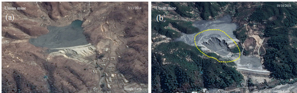
Fig. 9. Tailing dam in 2014 (a) and 2016 (b) at the Unsan mine
