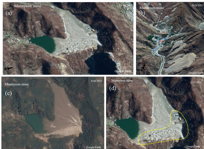
Fig. 8. Tailing dam (a) and waste rock dumps (b), Upper side of tailing dam in 2015 (c) and in 2017 (d) at the Mannycon mine.
