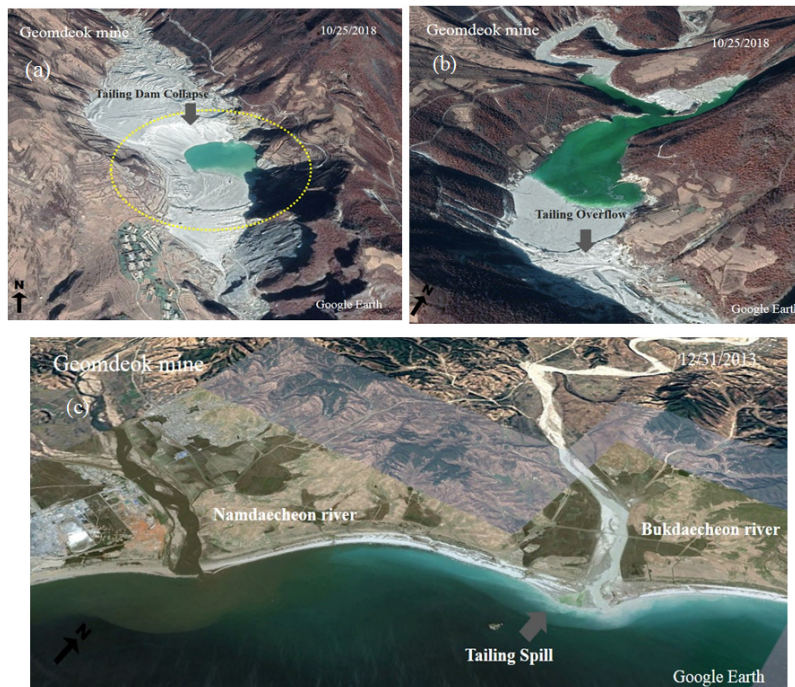
Fig. 3. Tailing dam failure (a), new tailing dam (b), and discharge of mine tailings to the East Sea (c) at the Geomdeok mine.
